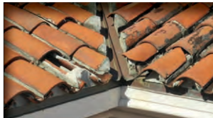
DAMAGED ROOF TILES
