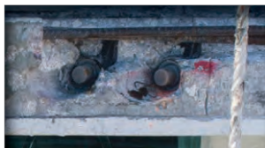
POST-TENSION CABLES
