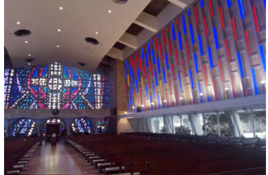
Church Sanctuary LED Lighting fixtures with 75% energy savings
