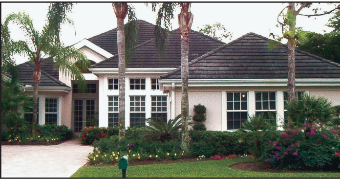
Before treatment with Roof-A-Cide ®
