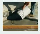
Sloping compound that provides a quick and easy way to fill in low spots on flat roofs and achieve positive slope to aid in proper drainage. The RoofSlope® compound is excellent for new construction as well as retrofit work, minimizing costs associated with fixing slope-to-drain issues.
