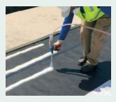
Pressurized foam adhesives specifically designed for adhering and securing roof tile, insulation and fleece back membranes across a wide range of substrates in both new and reroof applications. Polyset products use innovative polyurethane foam adhesive technology, providing a better finished project.
