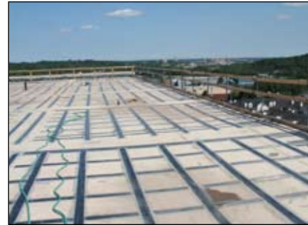
Examples of blast strengthening using Sika CarboDur plates and SikaWrap fabrics
