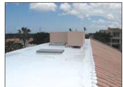
Seamless SikaRoof MTC liquid applied membrane. Note complex transition detail below
