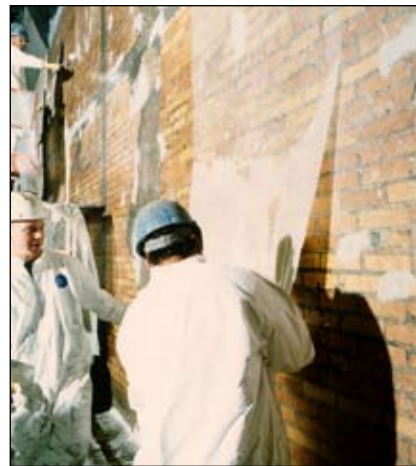
Glass fiber fabric being applied to strengthen unreinforced masonry wall.
