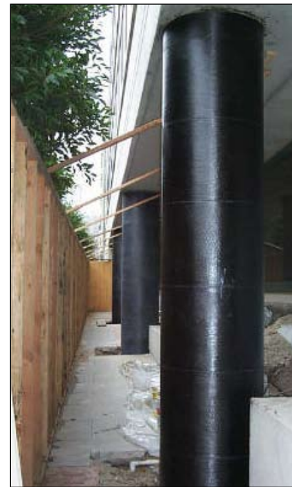
Seismic strengthening of columns with carbon fiber fabrics.
