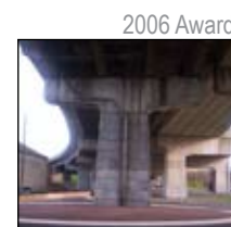
2006 Award Repaired in 1992 Silver Jubilee Bridge Repair
