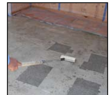
Application of Sika FerroGard 903 to a building (l) and a balcony (r)
