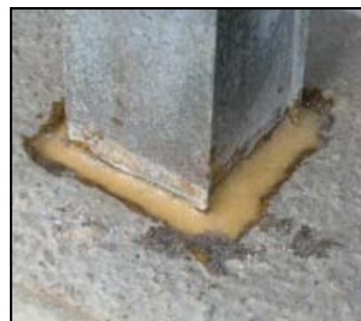
Sikadur 21 Lo-Mod with oven dried aggregate for rail post grout.
