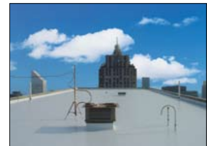
Seamless SikaRoof MTC liquid applied membrane. Note complex transition detail below
