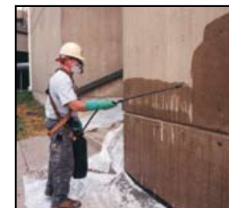
Application of Sika FerroGard 903 to a building (l) and a balcony (r)
