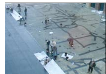
Plaza deck waterproofing with SikaRoof MTC Inverted
