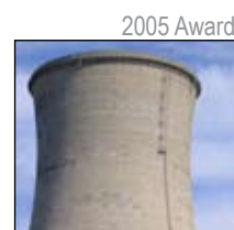
2005 Award Repaired in 1988-1990 Rehabilitation of Two Hyperbolic Cooling Towers
