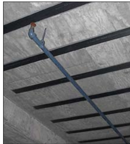
CarboDur plates used to reinforce a concrete slab.
