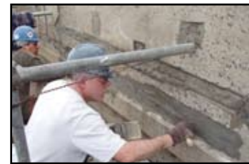
SikaTop 123 Plus used for vertical repairs.
