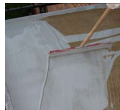
Application of Sikalastic base coat.
